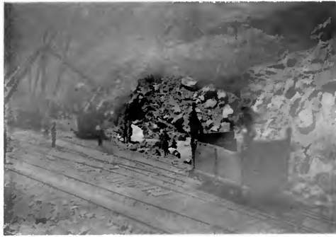
JACOBY CREEK QUARRY — LOADING THE CARS.
